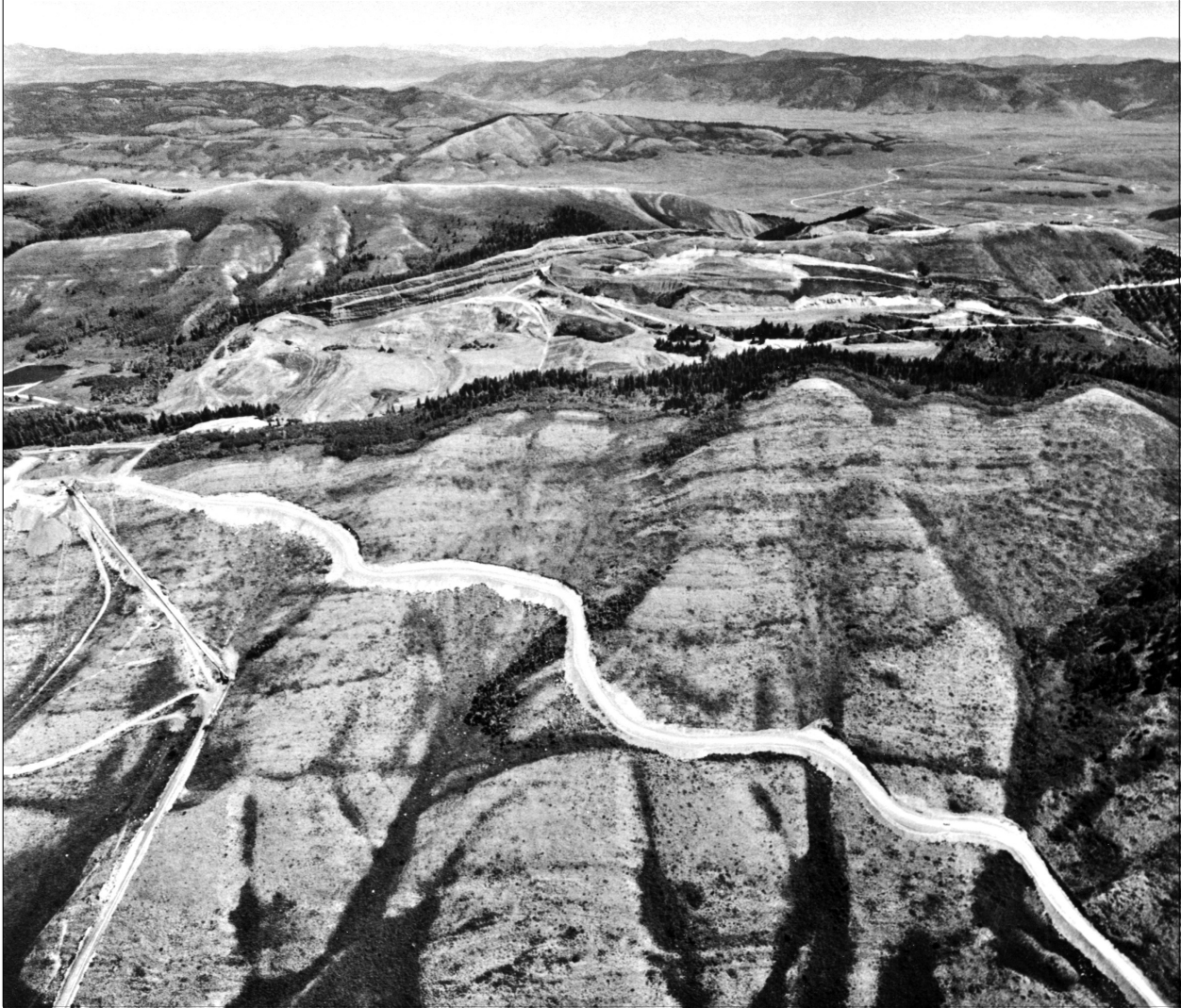
Figure 148. Mill Canyon Mine, view east, showing haul road and conveyor belt, July 18, 1984. BLM file photo.
